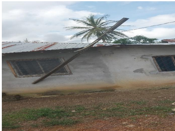
Service Drop on Plank
