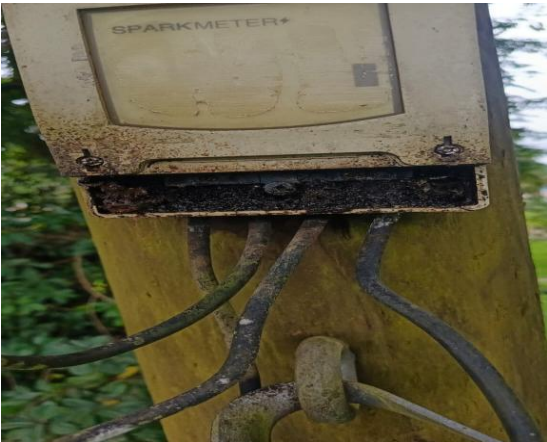
Damaged Meters
